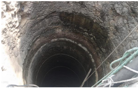
Plate 6.3 Field Photograph showing Open Well in Limestone
