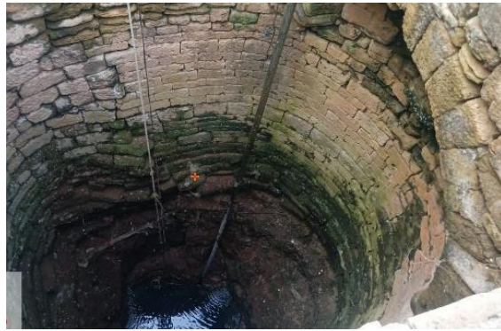
Plate 6.2. Field Photograph showing Open Well in Fractured Basalt. Block Una, Gir Somnath District
